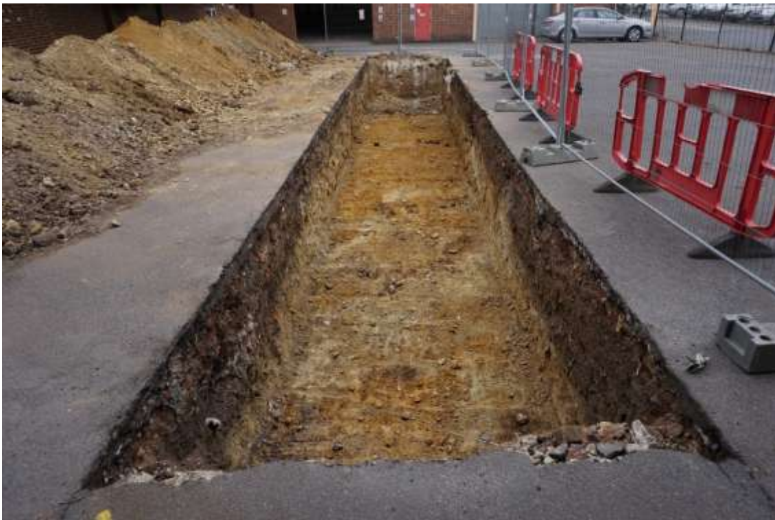
Plate 6. Trench 3 (looking E)
