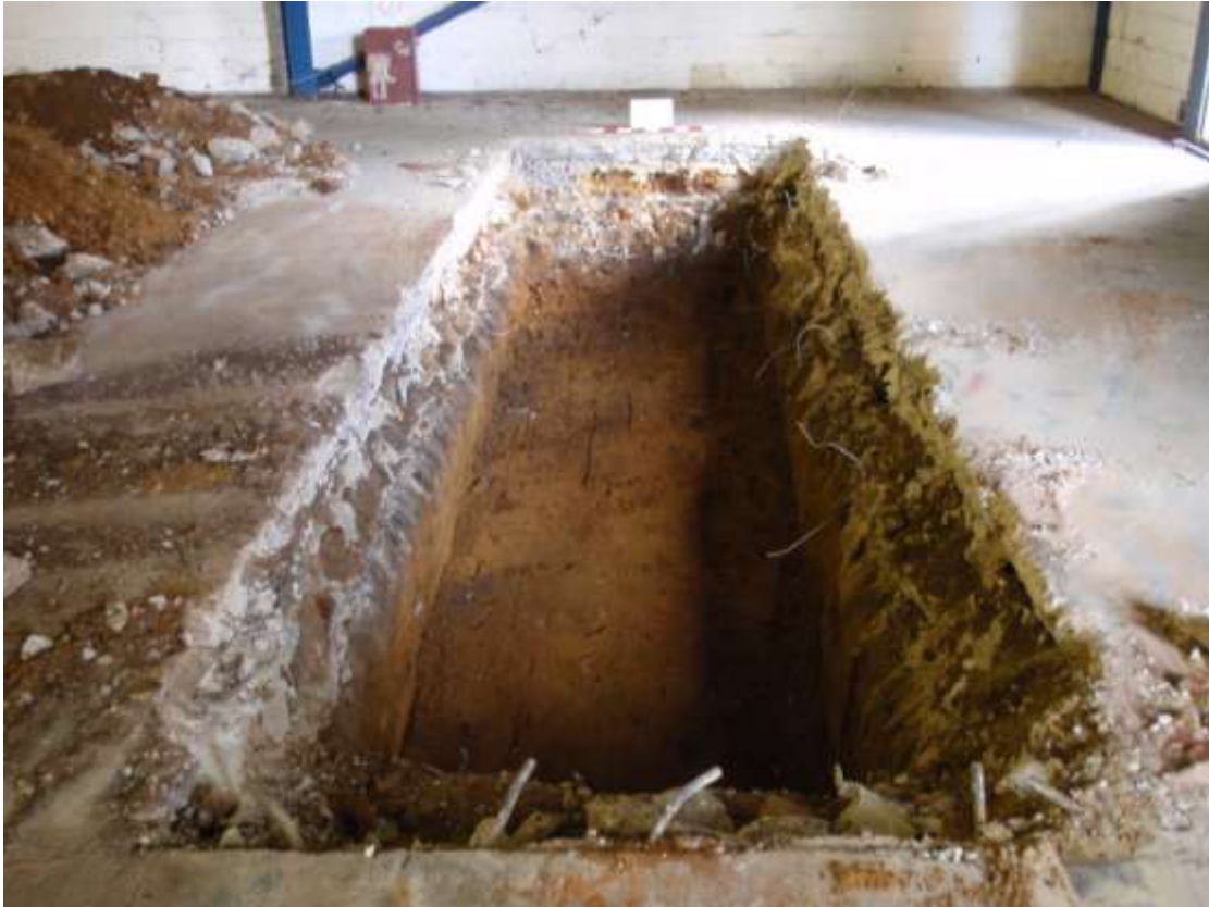
Plate 4. Trench 2 (looking NNE)
